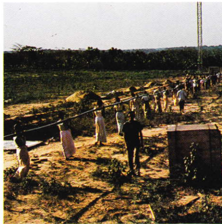
Laying the transmitter cable to the antenna – one example of many tasks that can be handled by local personnel.
